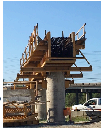
Photo Right: A steel cage sits inside of the pier cap form. An end piece will be added before concrete is pumped in and around the cage to shape the pier cap.
