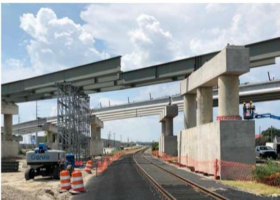
**Above:** Thick concrete crash walls are being constructed around all of the columns adjacent to train tracks.
