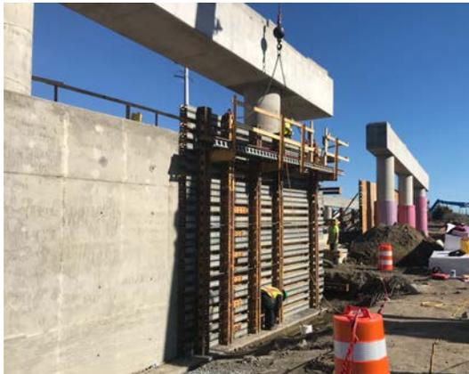
*Picture Above: Once concrete is cured and formwork removed, the project's first crash wall is revealed along eastbound Meeting Street.*
