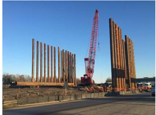
*Picture Above: By the end of February these pipe piles had all been driven 90 ft into the ground north of the Meeting and Spruill split.*
