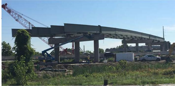
**Photo Above: Lines of girders over I-26 for a new ramp from I-26 EB onto Meeting Street.**
