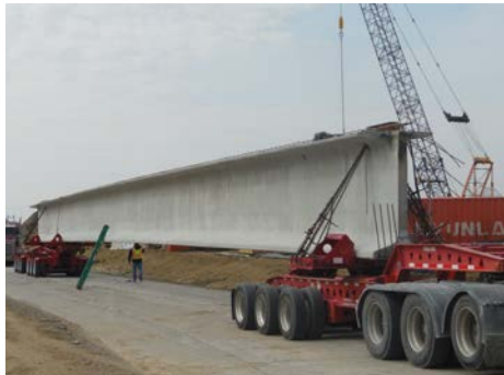
While this photo is not on our project, it does depict a concrete girder similar to the ones that will soon arrive for the new Meeting Street ramps on and off of I-26 and the mainline.
