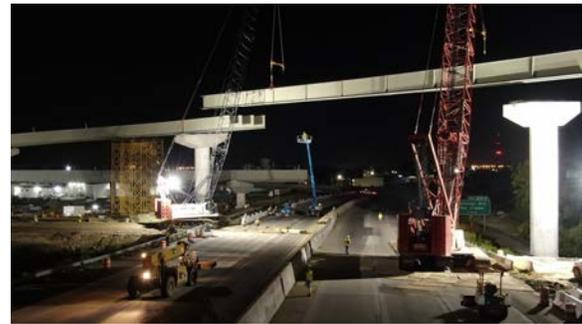
Thanks to team member Brad Chavis for the three drone photos. (top) Setting down the first set of girders over I-26 for the new ramp from I-26 Eastbound onto the Port Access Road. (above) Cranes work together to place girders in July for the new ramp from the Port Access Road onto I-26 Eastbound. (left) All of the curved girders are now in place over I-26. (below) An aerial view of the Port Access Road Project in July.
