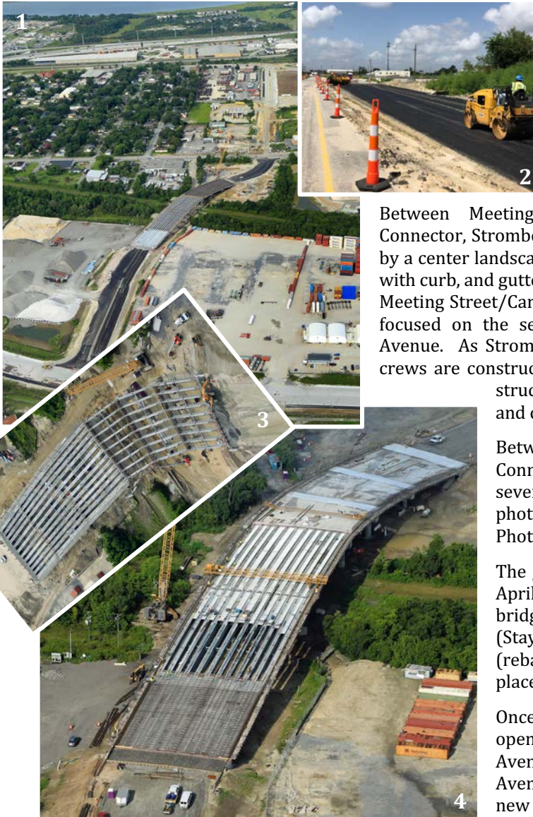
Photos: 1.) A July 2021 aerial photo of Stromboli Avenue from the new Bainbridge Connector Road at the bottom of the picture to Spruill Avenue at the top 2.) Placing the asphalt base layer for a wider Stromboli Ave. between Spruill Avenue and Column Street 3.) The new Stromboli Bridge in April 2021 4.) The Stromboli Bridge in August 2021
